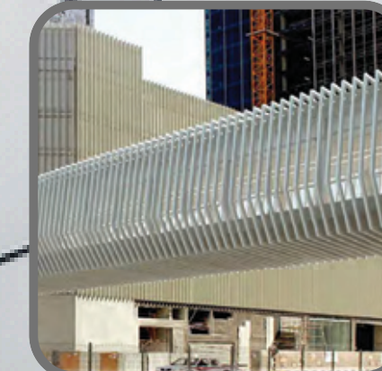
ACCESS FOOT BRIDGE TO AL RAYAN COMPLEX
