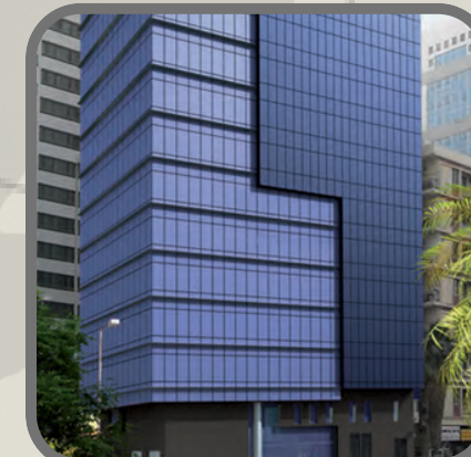
KHALIDIYA TOWER ABUDHABI ISLAND
